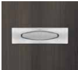
Anti-ligature features include inset pulls, continuous hinges and J-Bar in wardrobe
